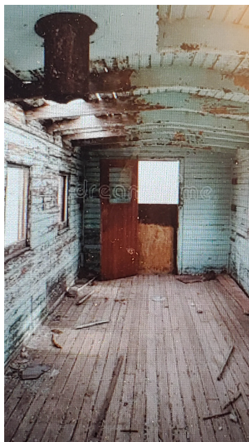
Caboose interior before rehab.
