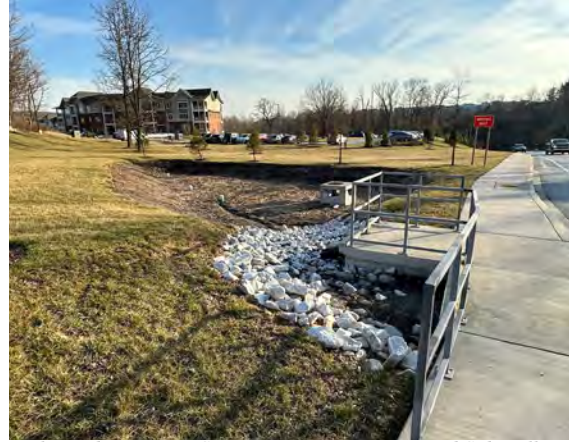
York Road Frontage: Stormwater Management and Sidewalks
