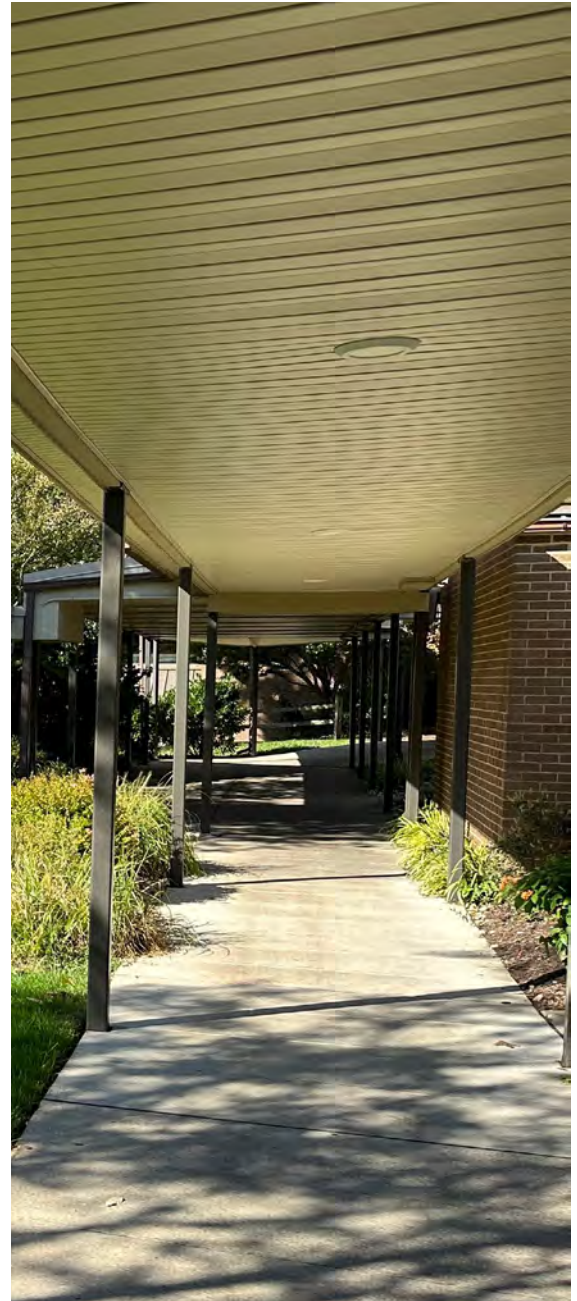
View of Garden Homes Covered Walkway
