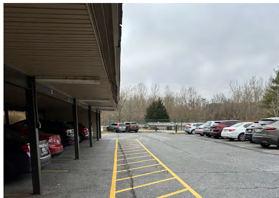
2 View of Zebra Stripe Painted Zone behind Parked Cars
