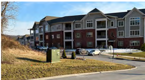
3 Infrastructure limitations at Copper Beech Lane intersection
