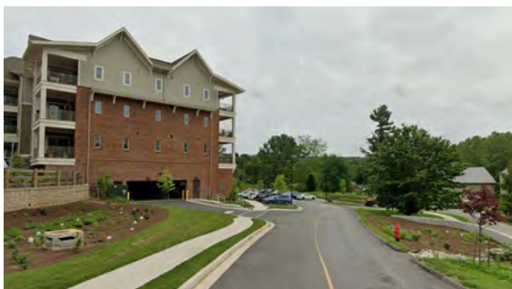
4 Exposed garages and young landscape
