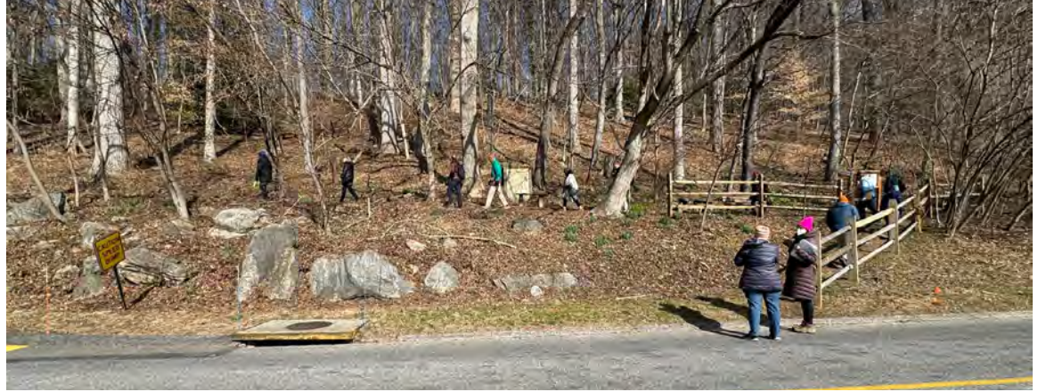
1 View of Trailhead without Sidewalk Connection
