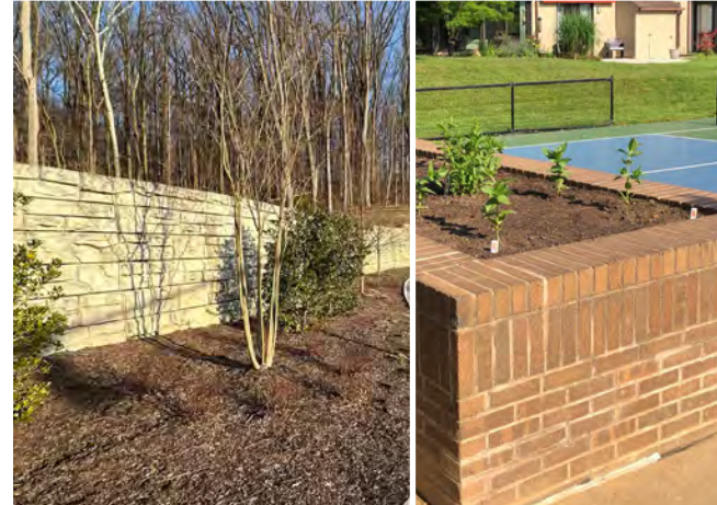
Views of Existing Walls and Fences
