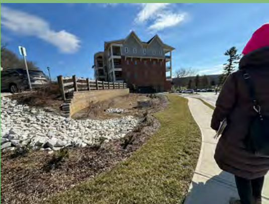
Infiltration (Bioretention adjacent Hillside Homes)
